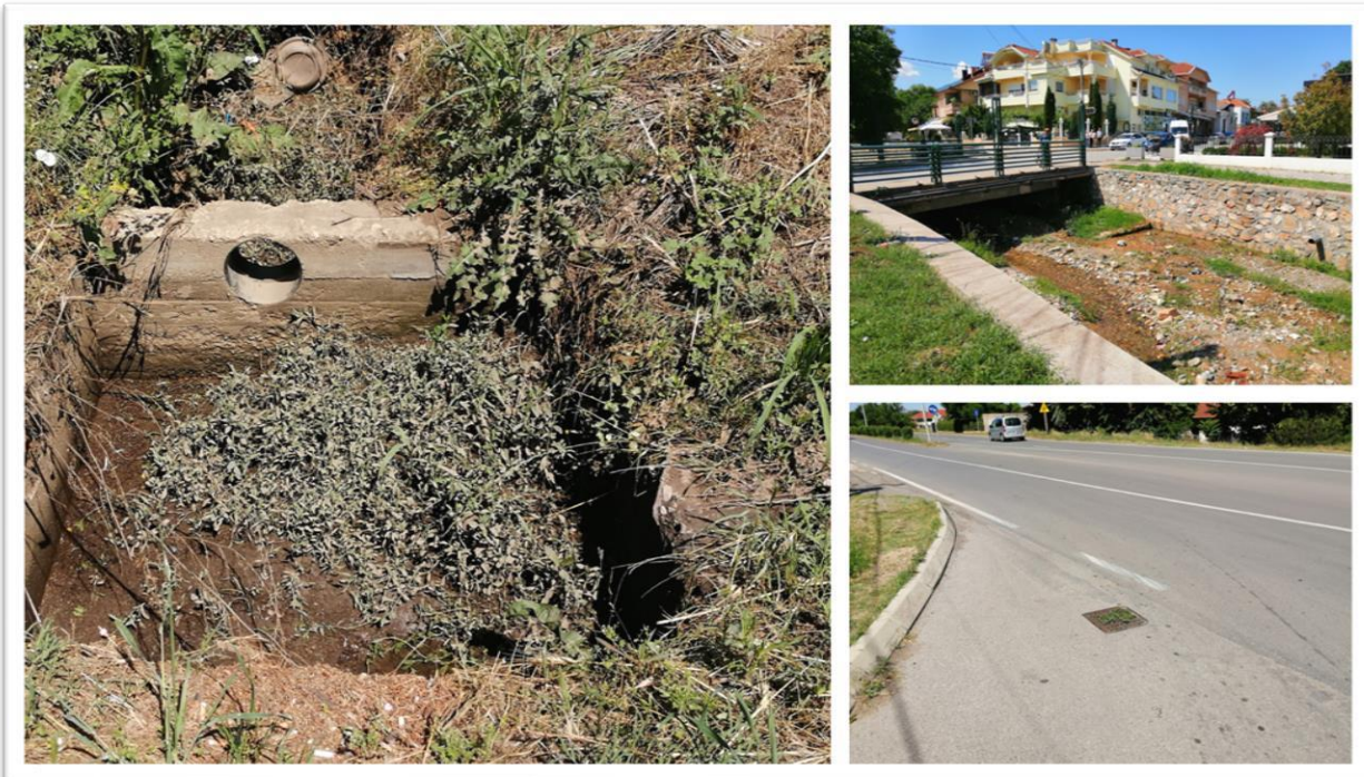
38. Figure: It can be seen that neither the existing drainage system, nor the riverbeds, nor the canals have been cleaned in drainage system of Vinica. Source: Self-made pictures
