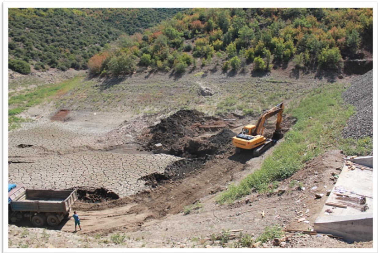
44. Figure: Development of pond for water drainage and retention outside Polog. Source: [26 – undp.org]
